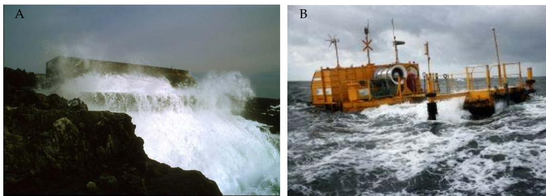
Figure 5.4. Examples of oscillating water column devices: A) © VHW 2012. The Limpet™ Islay power plant, Scotland, UK. B) © OE 2012. The OceanEnergy Buoy™.
