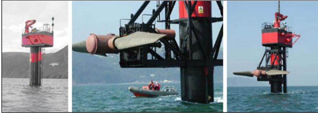
Figure 4.6. Seaflow installed off Lynmouth, Devon.
