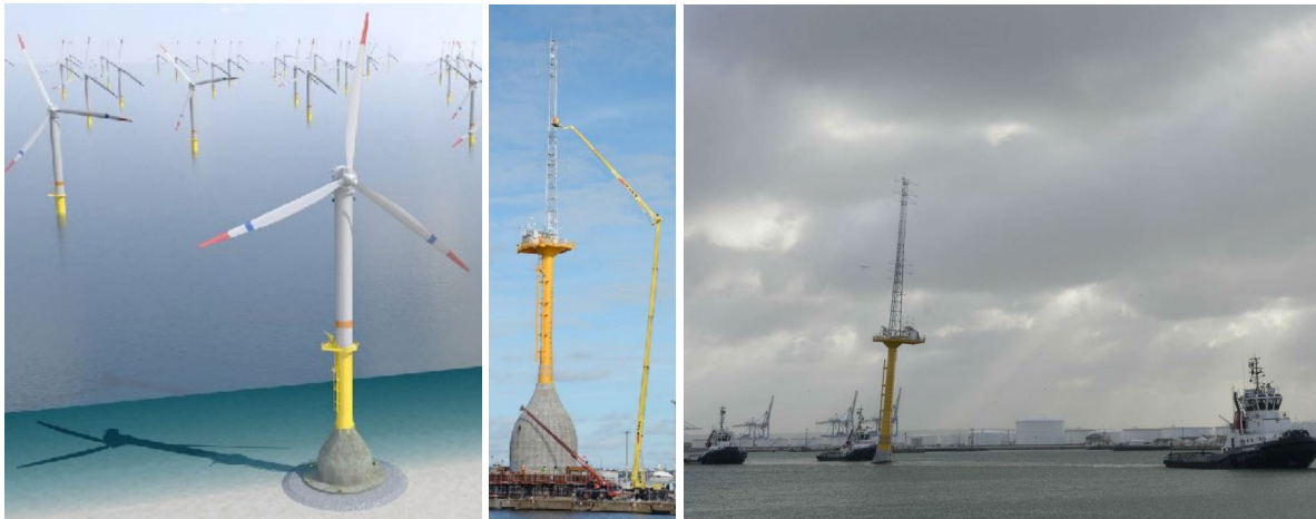
Fig. 12. Cranefree gravity base foundations: concept for an OWF using gravity base foundations (left). Construction of a foundation with a metmast in Fécamp, France (middle). Towing the metmast and its foundation to sea (right). © Seatower A/S.
